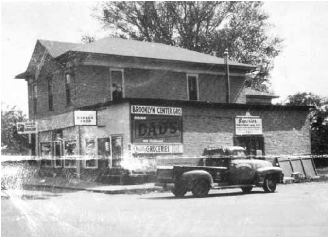
The Howe Store, located at what is now 69th Avenue and Brooklyn Boulevard.
